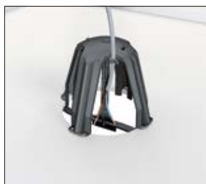
2. Push the spikes into the plasterboard to prevent shifting and disconnect the tool.
