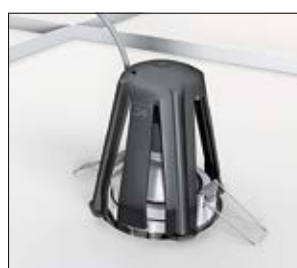
3. Start the installation of the downlight in a safe way.
