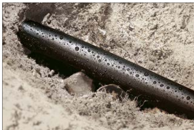
TREDUX HA47 - application below ground.
