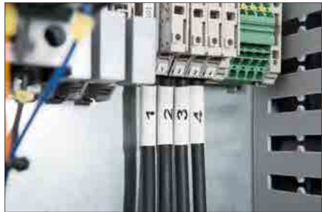
TLFD DS shrinkable markers for more safety and clarity in the switchboard.
